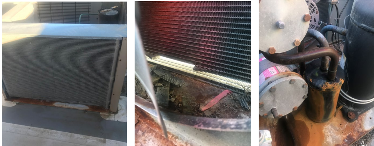
Photos above show the freezer condenser unit that is still functioning (limping along).
