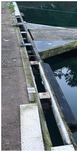
Left Photo – Dock finger re-attached (diamond-plate cover still off). Center Photo – Diamond plate back on. Right Photo – New pile hoop installed.
