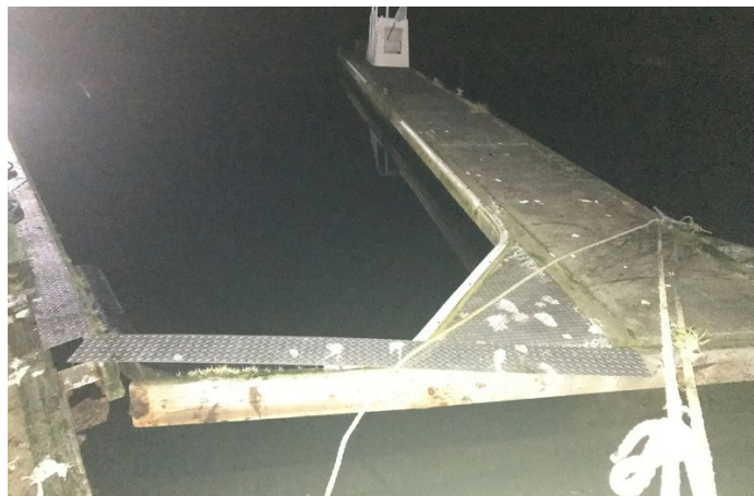
Photo on the left – Port Security reported the dock finger breaking loose at the start of his shift on Monday, January 19, 2026. Photo on the right – Dock finger broken loose at 7:00 p.m.
