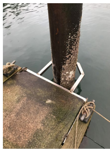
Left Photo – Dock finger re-attached (diamond-plate cover still off). Center Photo – Diamond plate back on. Right Photo – New pile hoop installed.
