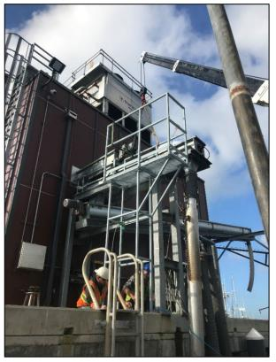
Charleston Maintenance Operators Dwayne Temple and Jeremy Beard fabricate and install a platform and ladder to allow access to the Ice Delivery System at The Charleston Ice Plant. Occasionally, the conveyor or chute plugs up requiring Charleston Maintenance Personnel to have to get a ladder to access it and clear the plug up. This will allow easier and safer access. Cost of the materials was minimal due to salvaged and repurposed walkways, handrails, and ladders from T-1.
