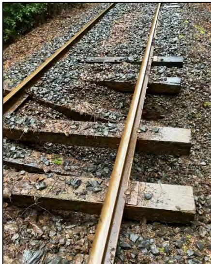
(Culvert failure, causing washout near Ada)
