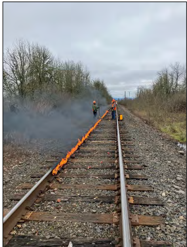
(Rope burn to warm up rail to stretch it for repair)
