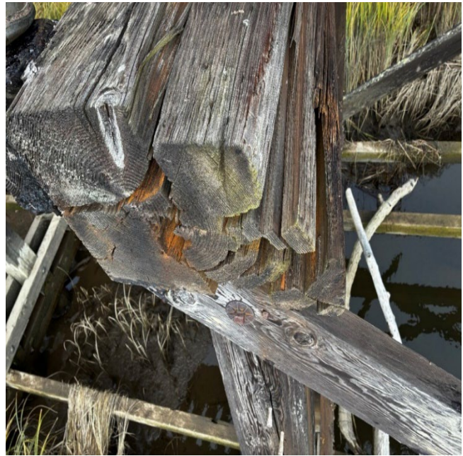
(Failed cap at bent 133, MP716.4)
