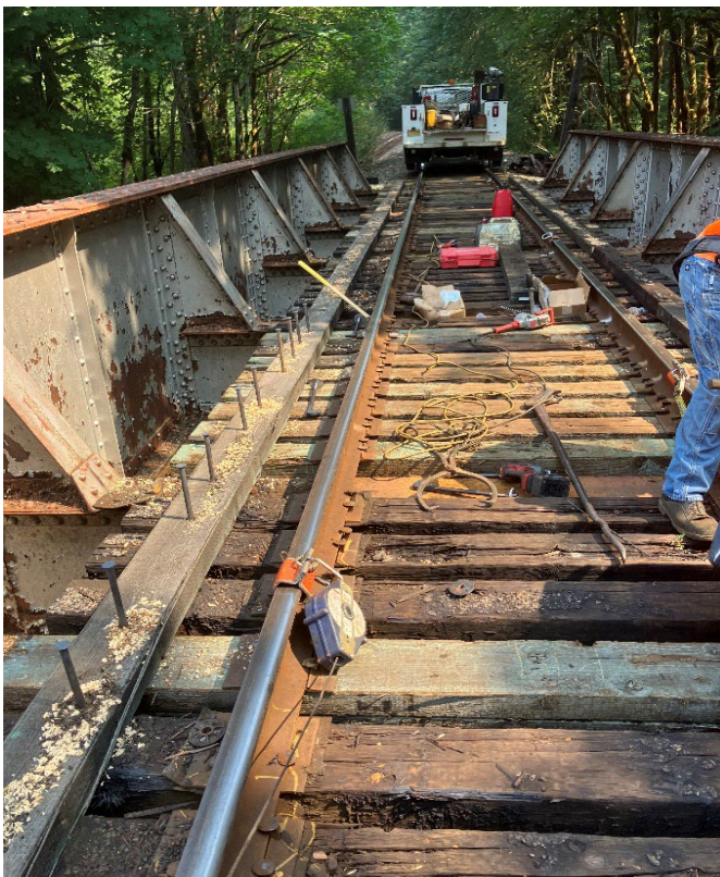
(Bridge Tie and Guard Timber replacement MP 683.4)
