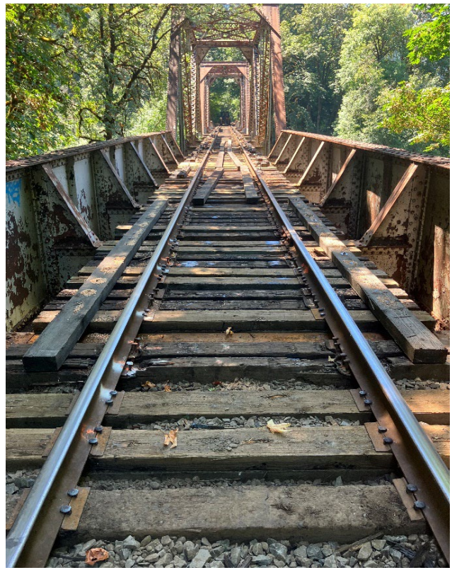
(Bridge Tie and Guard Timber replacement MP 683.4)
