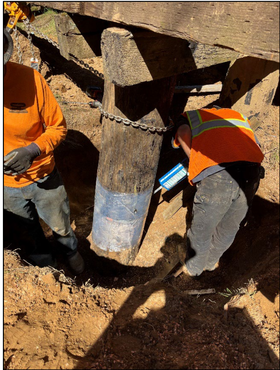
(“Posting” a failed piling)
