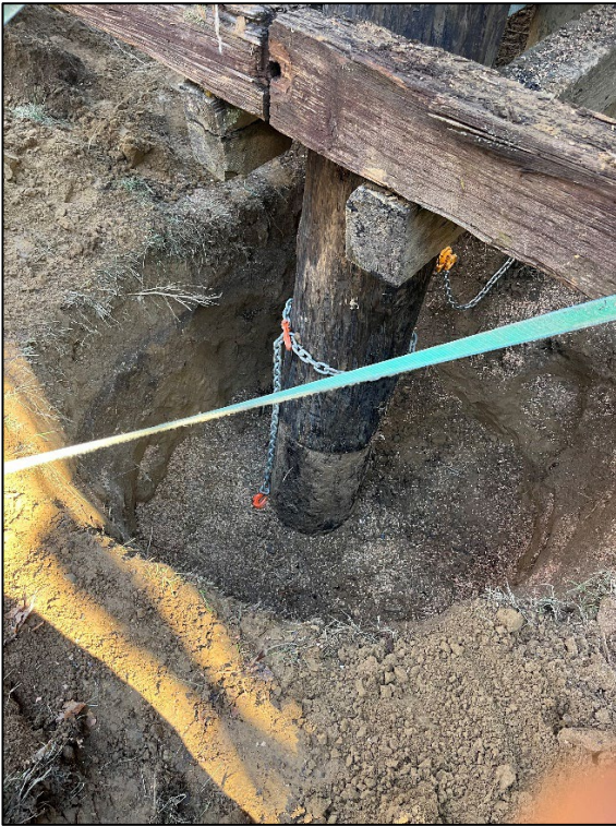
(“Posting” a failed piling)
