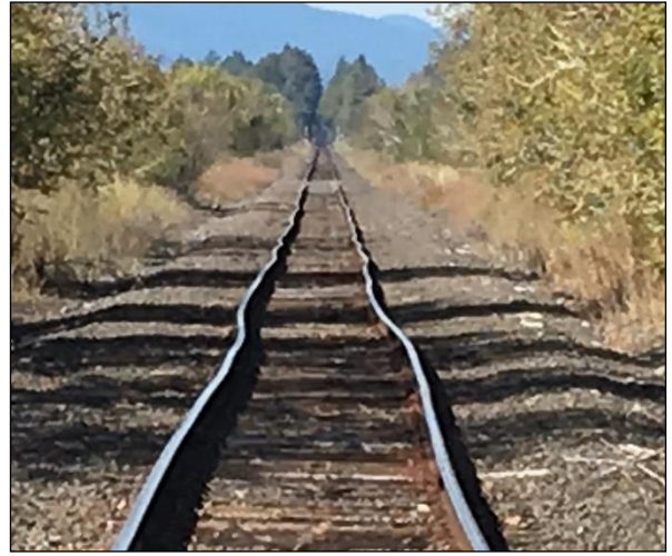
Figure 2: Track surface MP656.12
