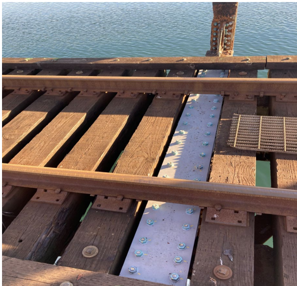
Floor beam strengthening and post replacement.
