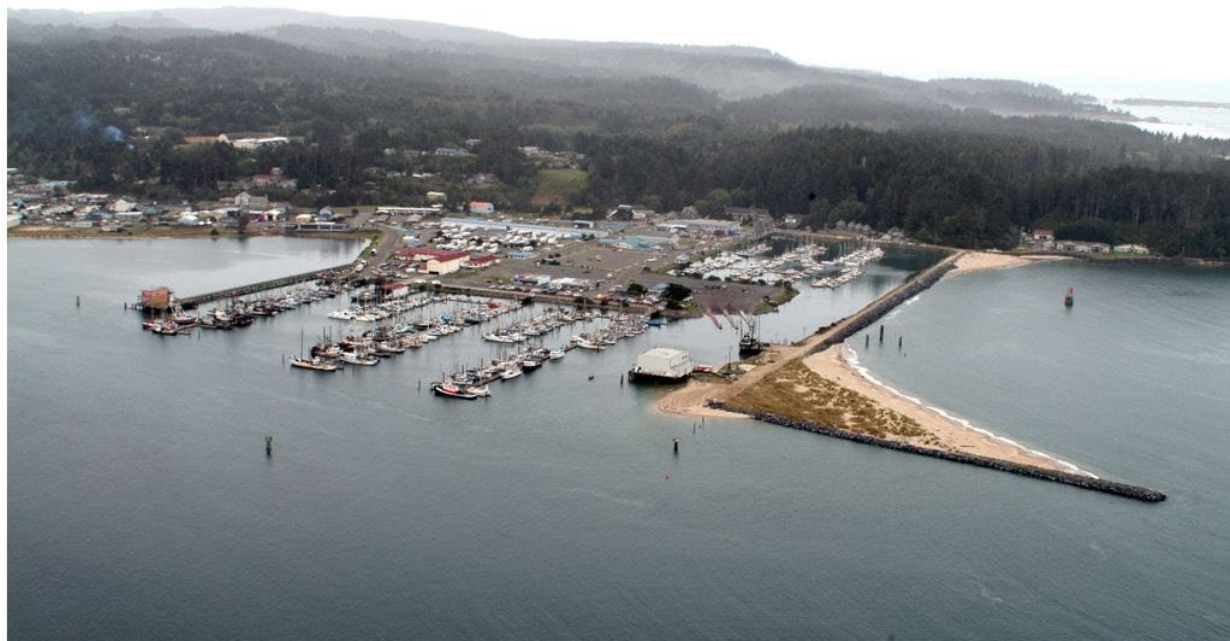
Figure 2-17: Charleston Marina and Breakwater, Looking West
