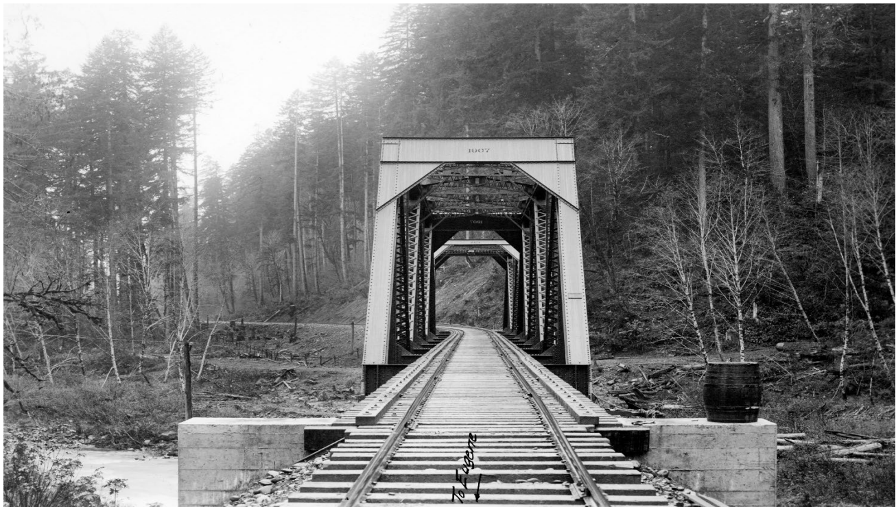
(Bridge over the Siuslaw at MP 691.05, 1914)
