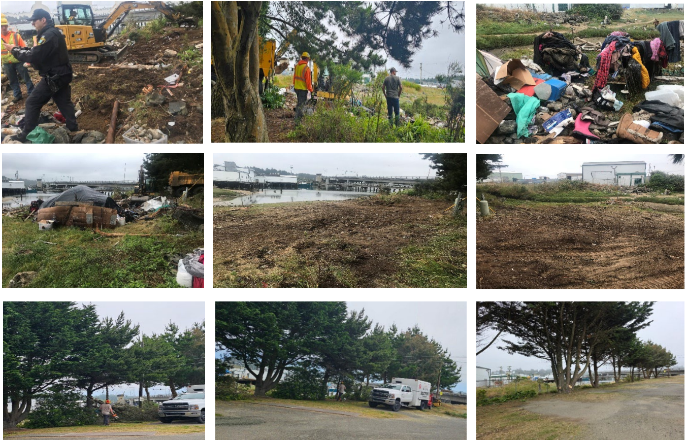
The photos above are before, during, and after the clean-up.
