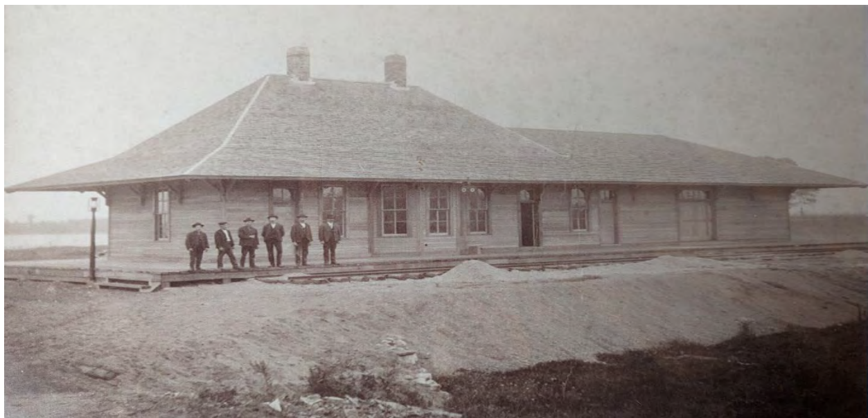
(Rail being laid, North Bend passenger station 1914)
