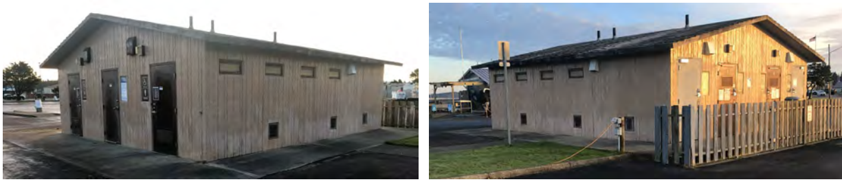
Above: The exterior of the Inner Basin Restroom.
