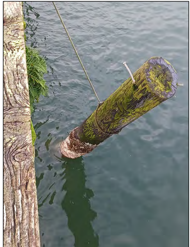
A broken wood piling that was removed during the 2023/2024 Piling Project
