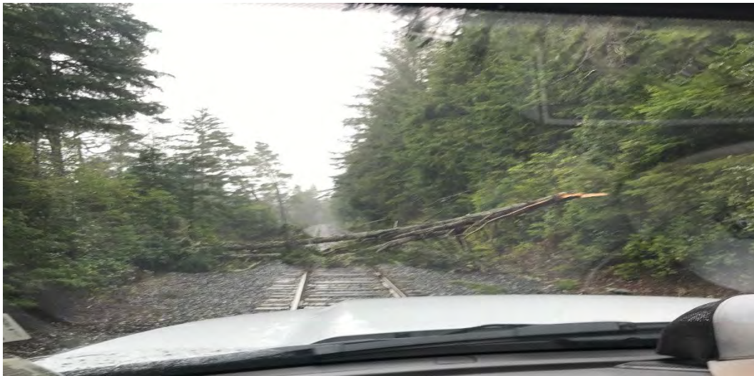
Track Inspection hazard.
