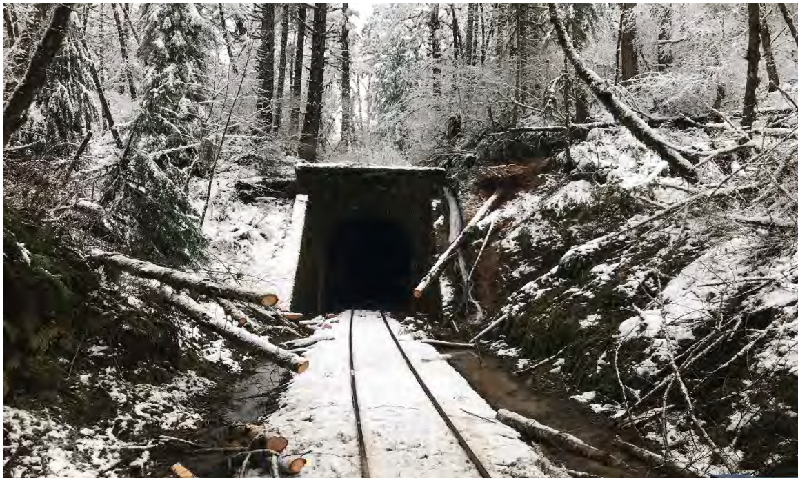
Trees cleared at Tunnel 14.
