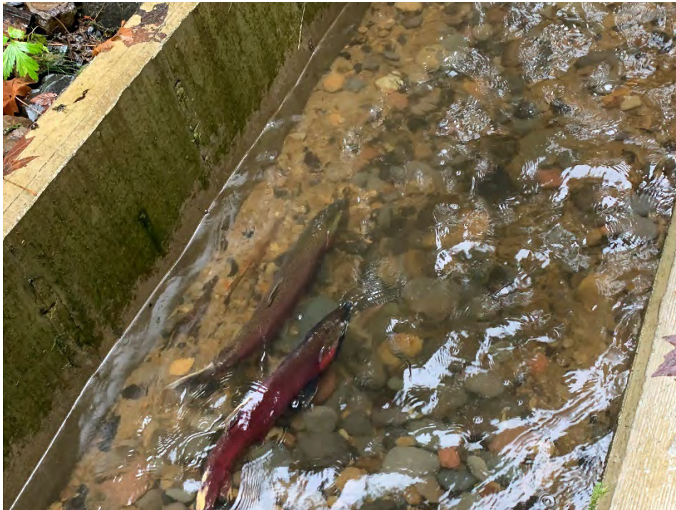
Tunnel 19 Salmon in culvert.
